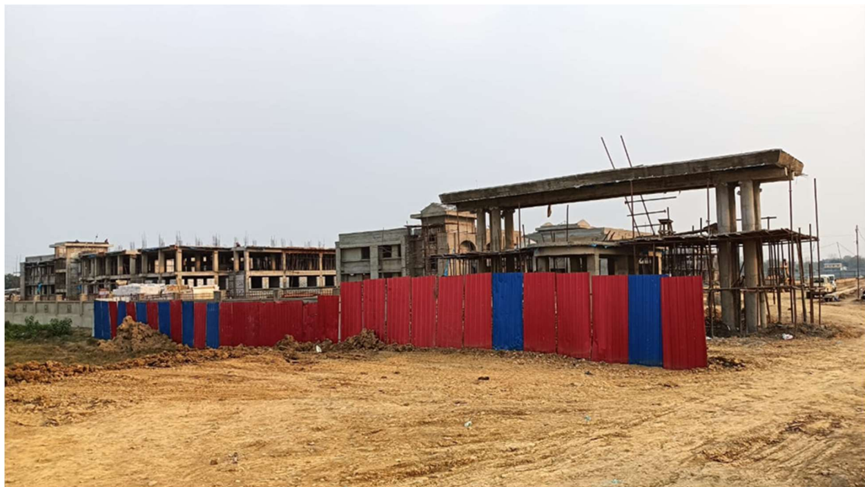
New University Gate under construction
