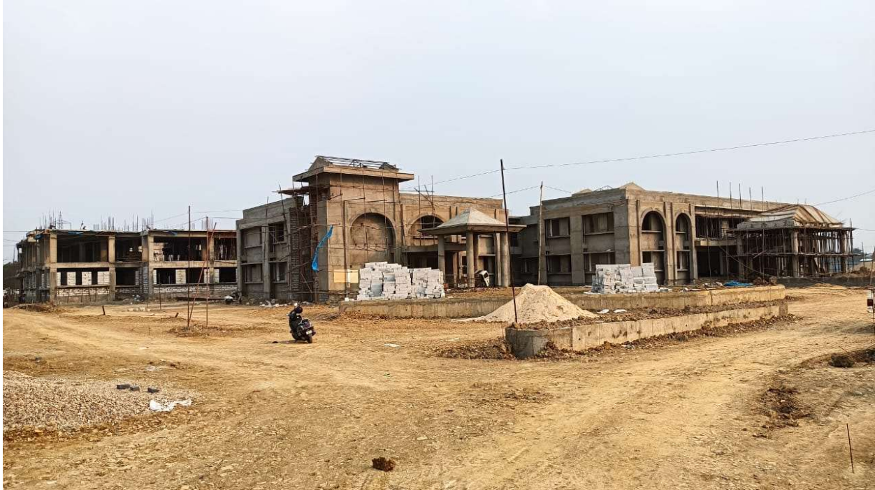
New buildings of Rabindranath Tagore University under construction
